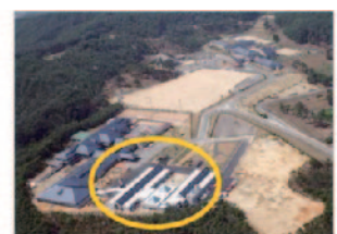
1989: The geriatric health care facility had been established
